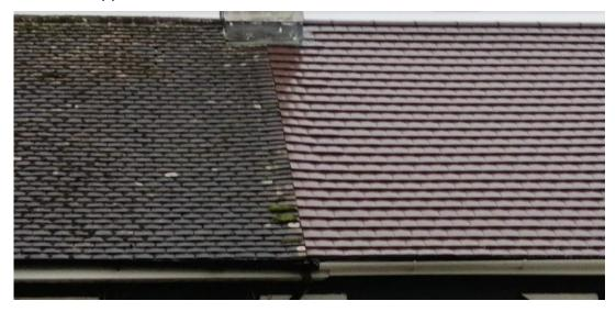
The original roof on the left has been fitted with a concrete granular faced plain, double lapped tile. The second (10 Duffryn Close) has a single lap, interlocking double plain tile.
