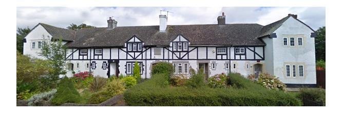
There are striking differences between the original double lapped tiles (left) and the cheaper single lap tiles (right at number 10).
